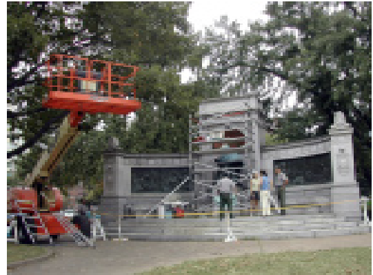
Renovation Crew at work
