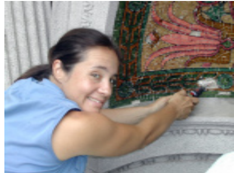
Kimberly Carter removing old grout
